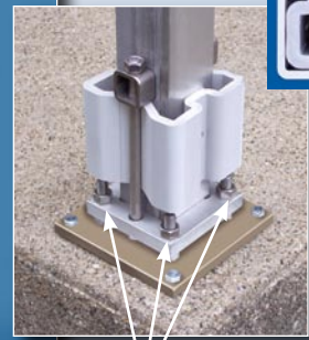
Angle Adjustment Leveling Bolts
