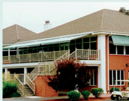
2ND STORY PATIO SEATING AREA AT GOLF CLUB
