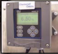
Automated Chemical Test Pretreatment chemicals are monitored and added automatically but titration is checked manually twice per shift.
